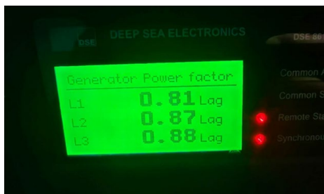
The power factor before the ESS was deployed
