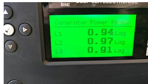
The power factor after the ESS deployment
